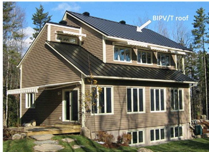
Figure 2.5. EcoTerra low energy solar demonstration house in Quebec, Canada (Chen et al., 2010)
