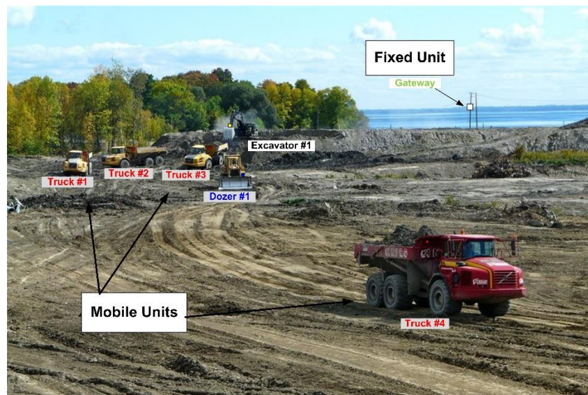
Figure 4-23: Conceptual deployment of Sensor Aided GPS Prototype
