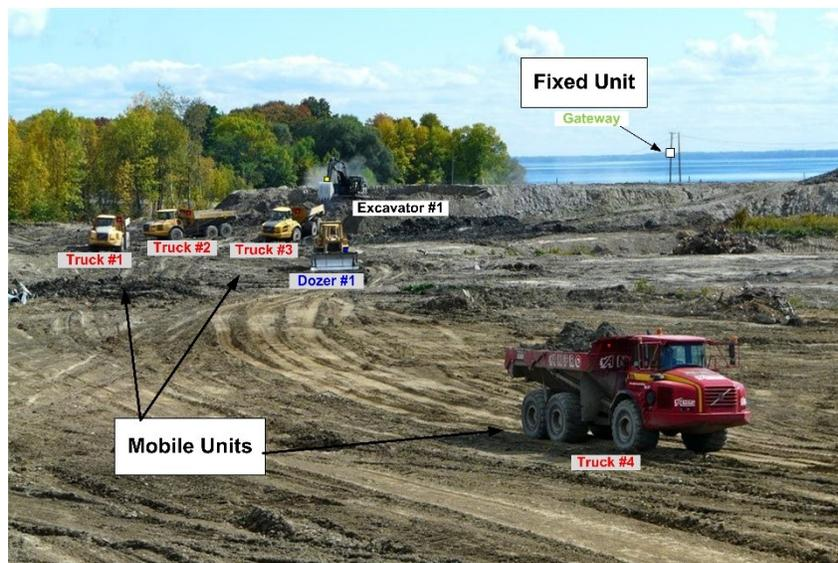
Figure 4-23: Conceptual deployment of Sensor Aided GPS Prototype
