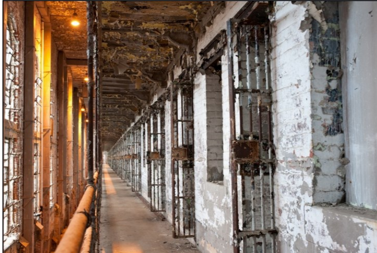
Figure 5. The west cell block of the Ohio State Reformatory
