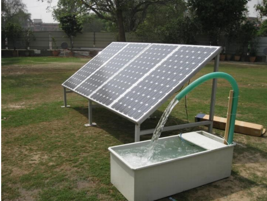
Figure 6.5: Solar panels provide enough power to run small pumps, and may eventually be able to provide power to efficiently drain large tile systems. Image taken from: http://belkomsolutions.com/?page_id=909
