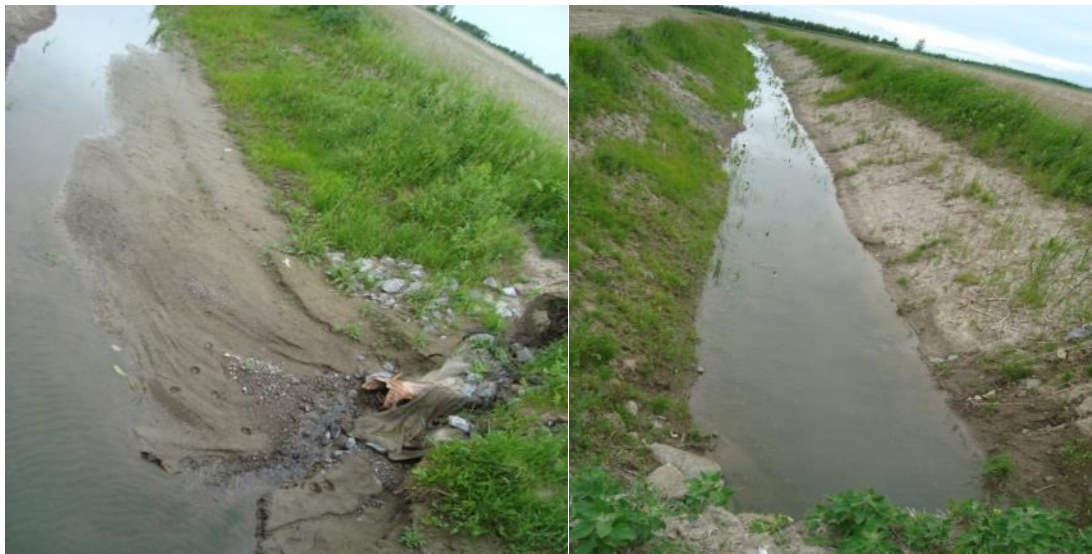
Figure 1.1: Clogged outlets (left) are a prime motivation to carry out dredging operations (right photo shows a recently dug ditch).
