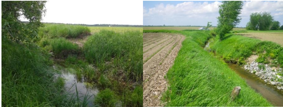
Figure 1.3: Bank failure due to erosion (left) and riprap applied to counter this phenomenon (right) in the des Fèves watershed.
