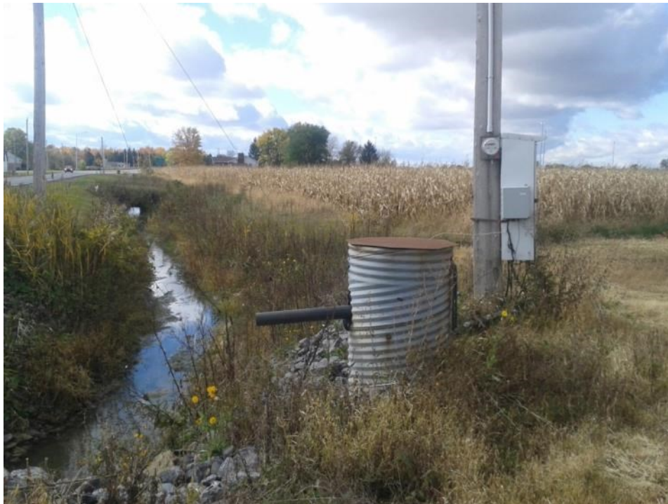
Figure 6.4: This electrical pump is located close to a road, where electrical lines are already present.
