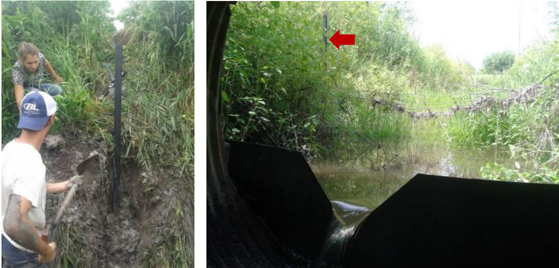
Figure 2.9 ABS pipe installation for a pressure transducer (left picture) and V-notch weir installed at a culvert – the ABS pipe can be seen in the back on the left bank (red arrow in the right picture).
