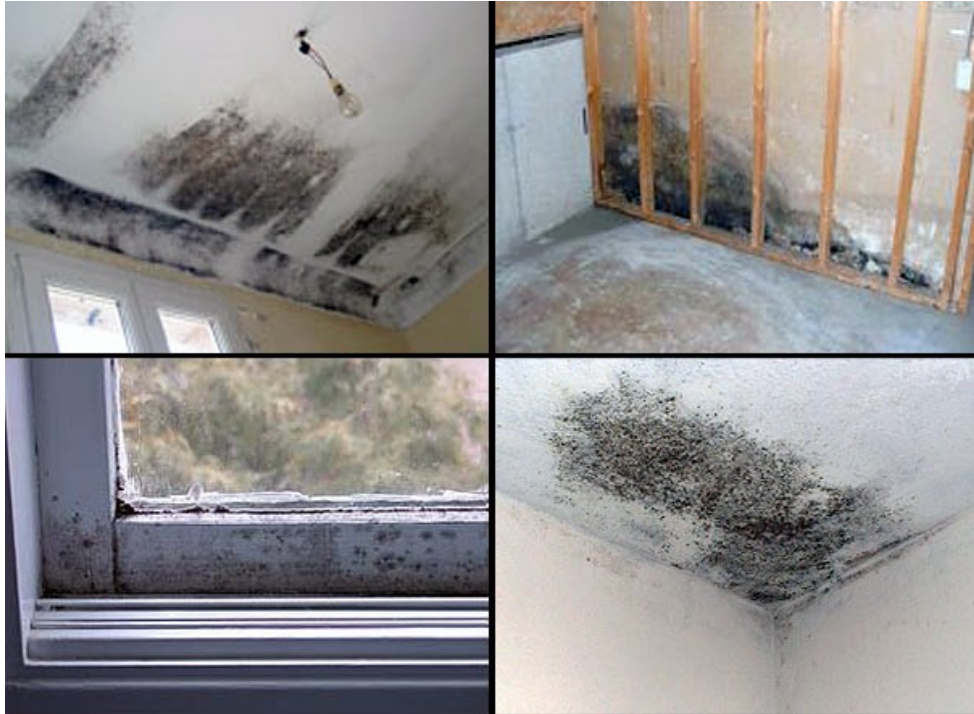
Figure 2.1 Mould formation caused by thermal bridges
