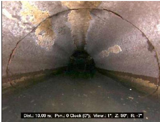
Figure 1.1 CCTV Caption of a Circumferential Crack Defect
