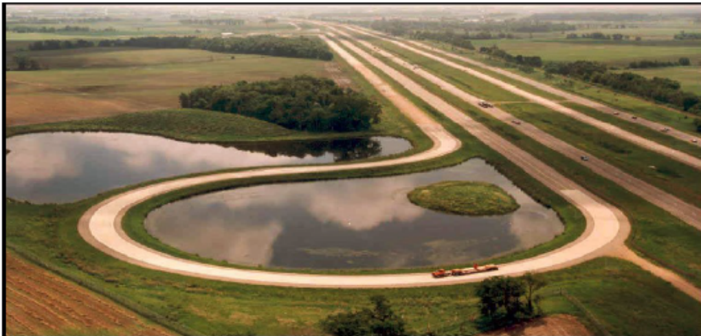
Figure (2-7) MnRoad full scale project, www.mnroad.dot.state.mn.us , 2000.
