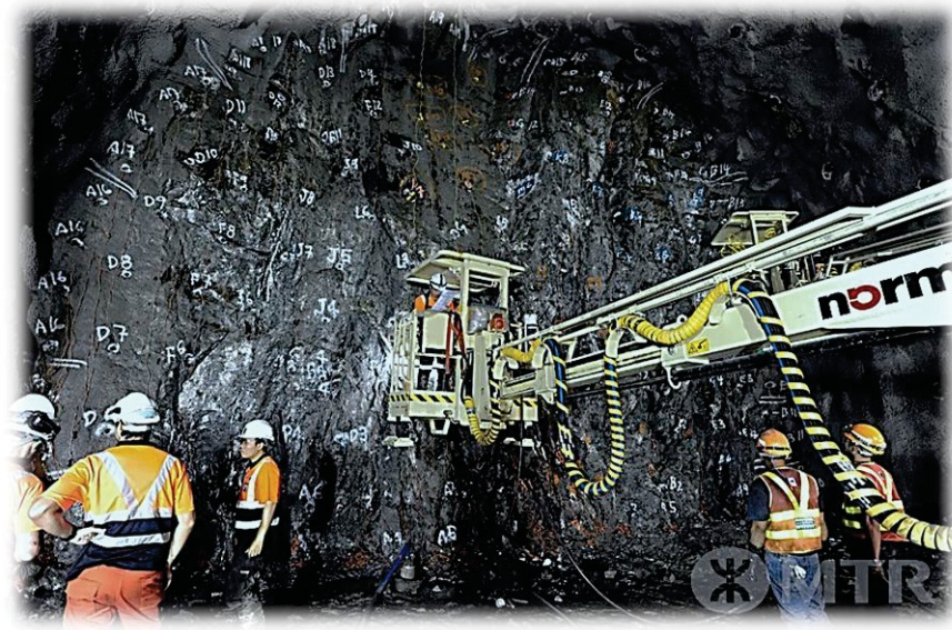
Figure 3. Qualified professionals are carrying out drill and blast works (MTR, 2013)
