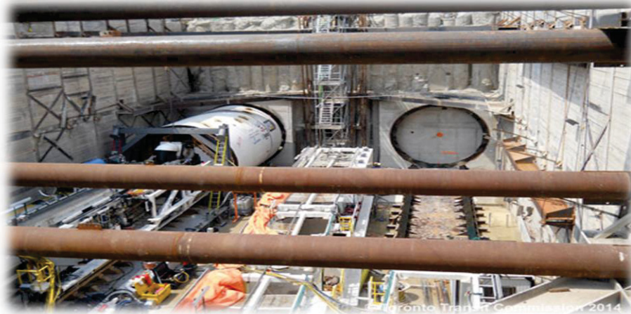
Figure 43 Downs-view Park Station Launch Shaft (Kiewit, 2015)
