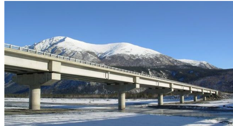
Fig. 3-9b Bridge #2 – with New Pier Cantilevers
