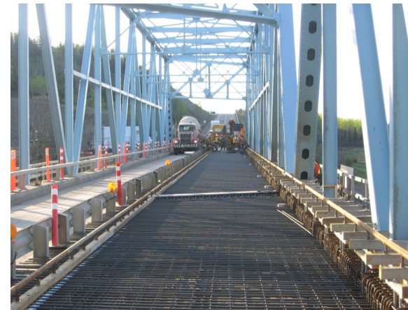
Fig. 3-9h Bridge #12 – Deck Replacement – One Lane at a Time
