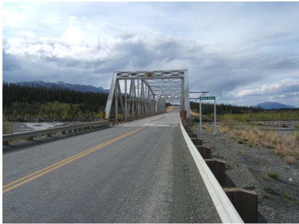
Fig. 3-9c Bridge #3 (Before 2009 Replacement)
