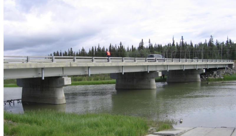
Fig. 3-9b Bridge #2 – with New Pier Cantilevers
