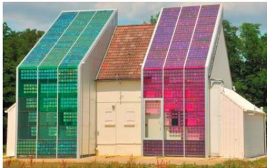
Figure 2.13: Prototype building envelopes installed on individual houses in Moret sur Loing, France (Gaillard et al., 2014a)
