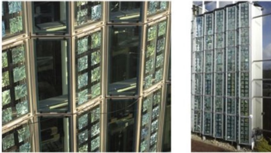
Figure 2.12: Prototype pleated PV double facade installed in Toulouse, France (Gaillard et al., 2014b)
