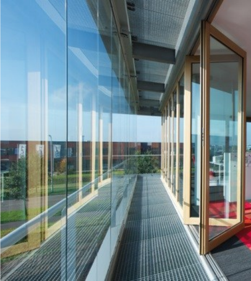
Figure 1.2: DSF implication in a new office building in Netherlands ( https://facadeworld.com/2014/03/15/solarlux-nijverdal/ )
