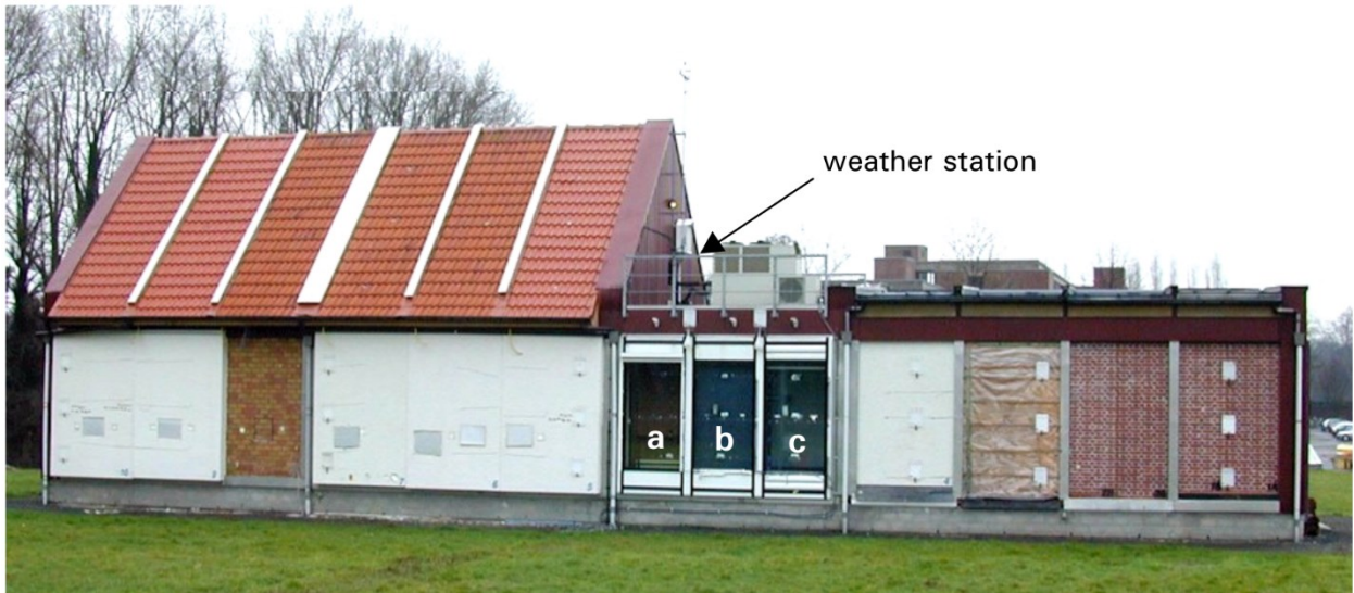
Figure 2.2: Vliet test building in Leuven, Belgium (Saelens, 2002).
