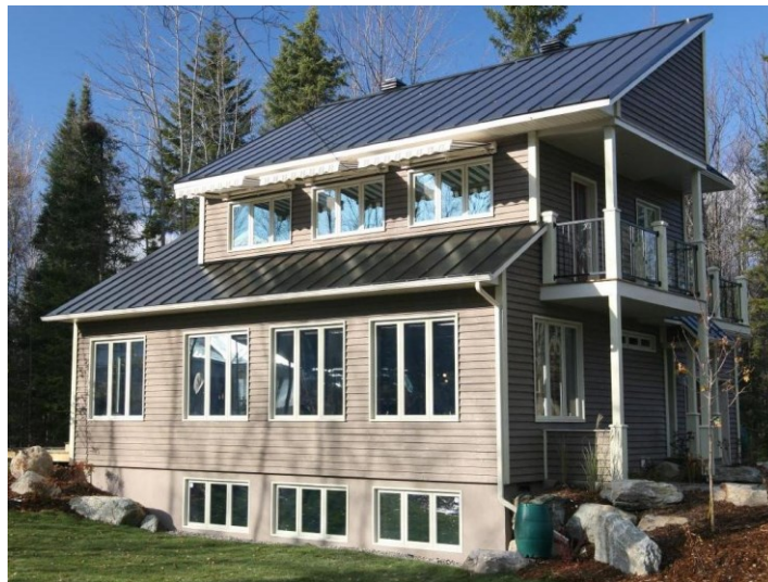
Figure 2.7: Eco Terra demonstration house (Chen et al., 2010a)
