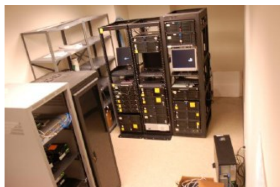
Figure 2-19 Full view of objects inside a room (CheckVideo, 2014)
