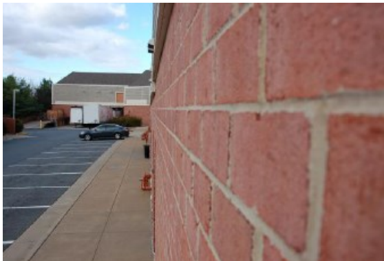
Figure 2-22 Placing the camera directly to the wall (CheckVideo, 2014)
