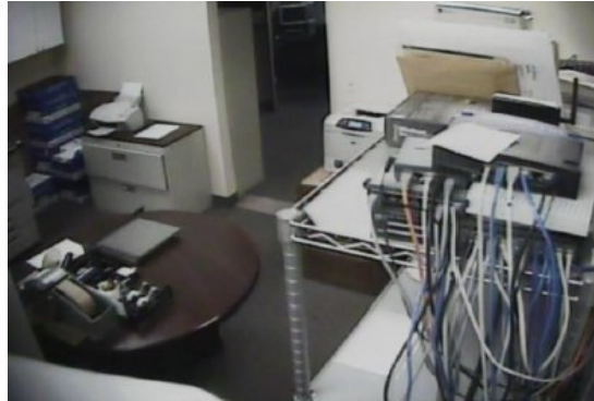
Figure 2-12 Object obstructing the camera view (CheckVideo, 2014)
