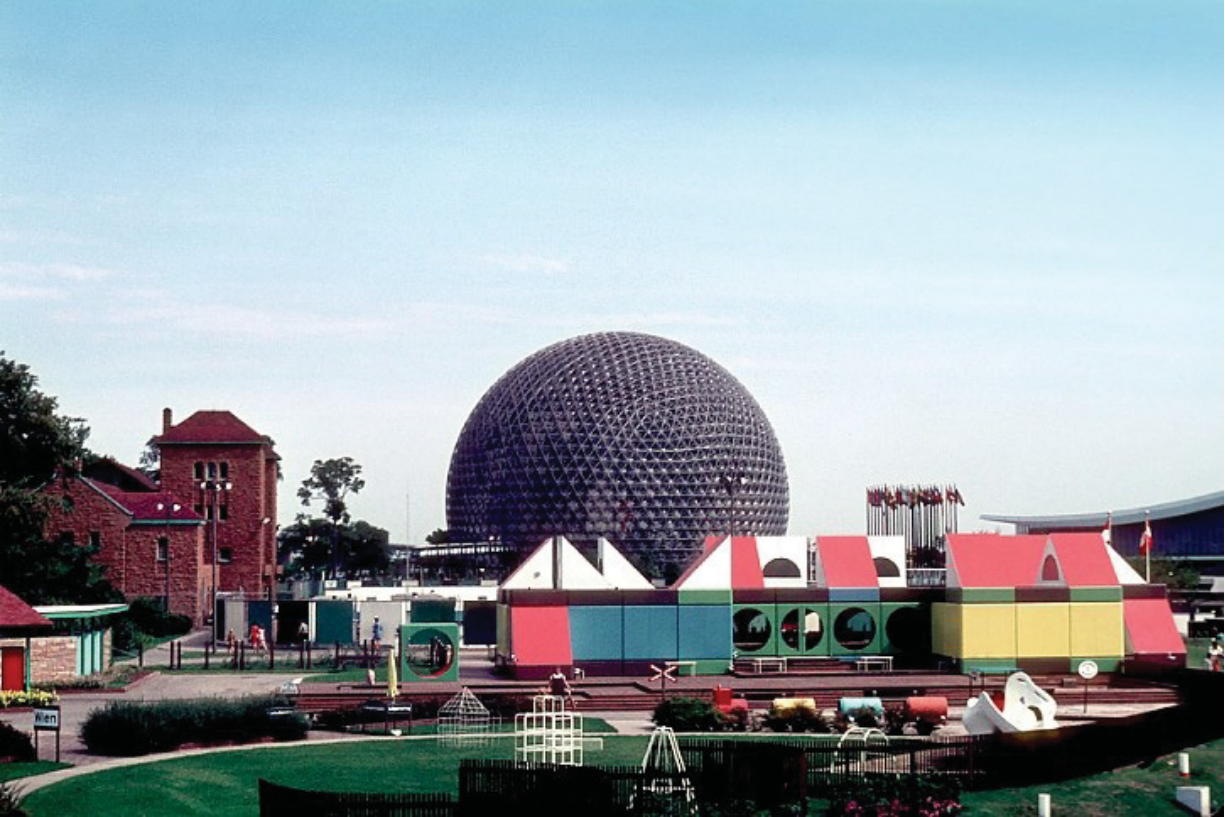
Figure 4. View of the play-yard and building of the Vienna Kindergarten at Expo 67. Bill Cotter. 1967. Photograph.
