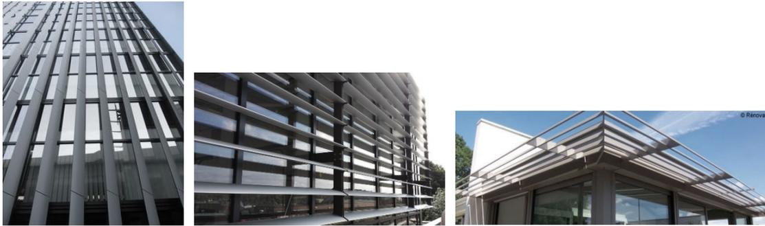
Figure A.3: vertical and horizontal exterior louvers (Bellia et al., 2014)
