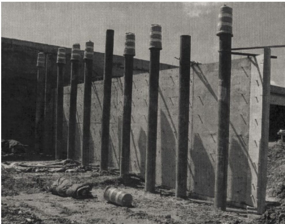
Figure 1.1.1 Pile foundations for a bridge overpass structure located nearby a retaining wall (Weaver and Youn, 2008)
