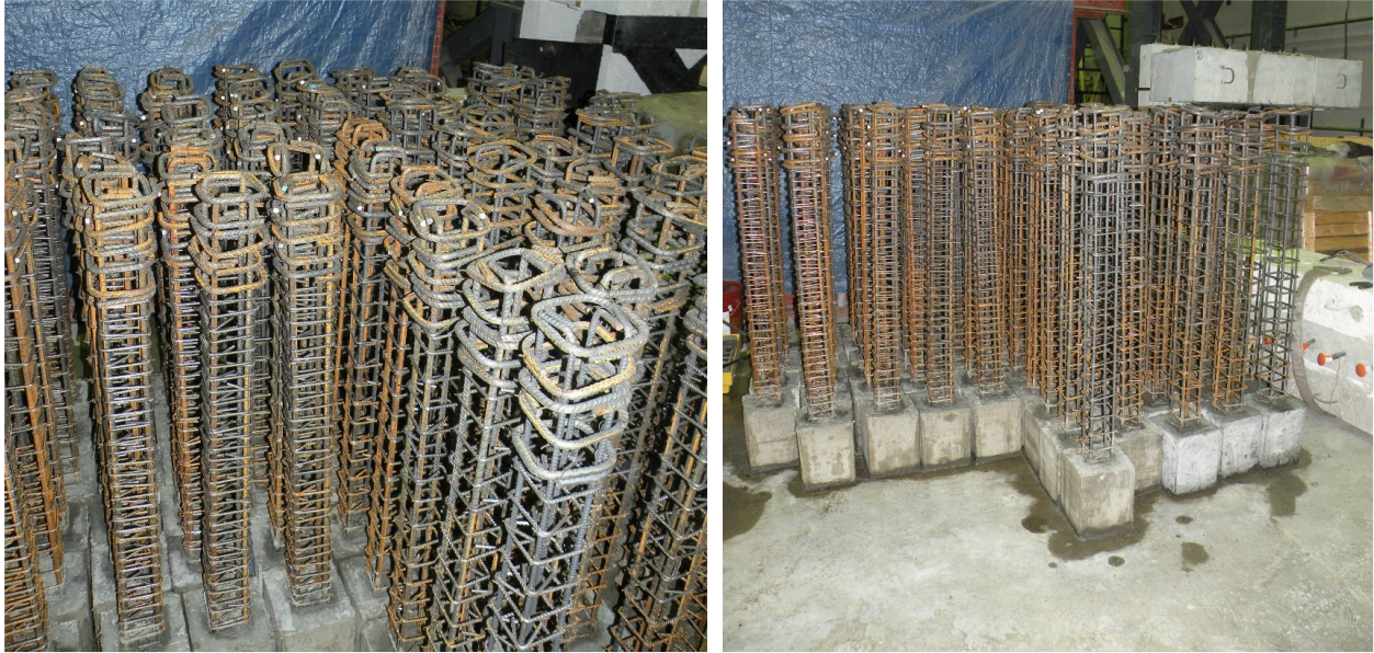
Figure A.11 Curing of the RC footing of the RMBE specimens
