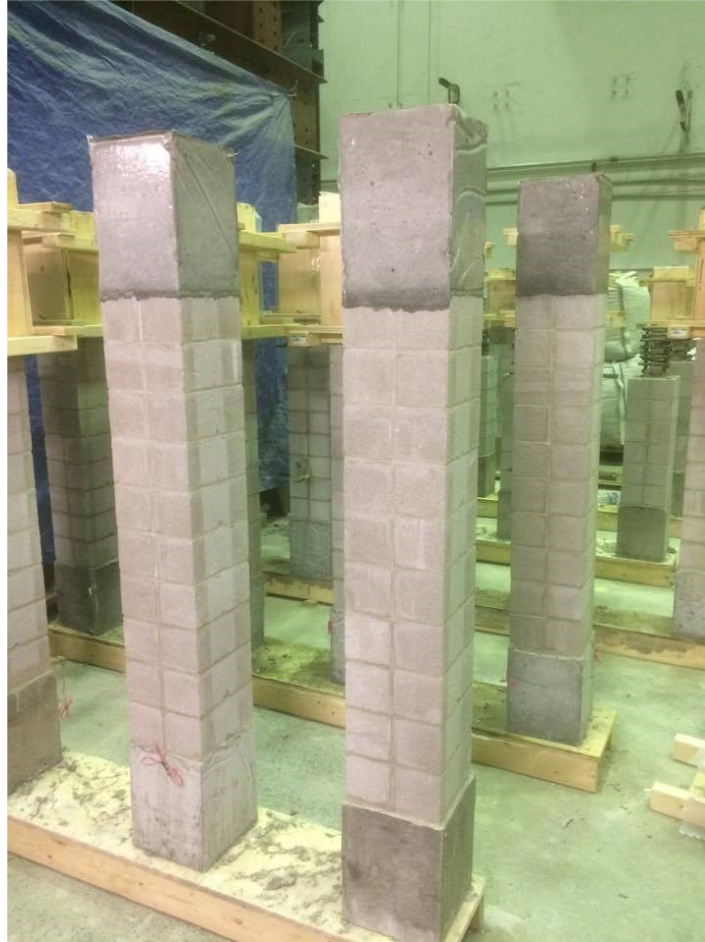
Figure A.20 Construction of the top RC footing
