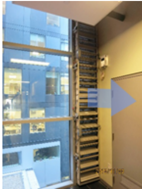
(c) Motorized inlet dampers allow the air into the building
