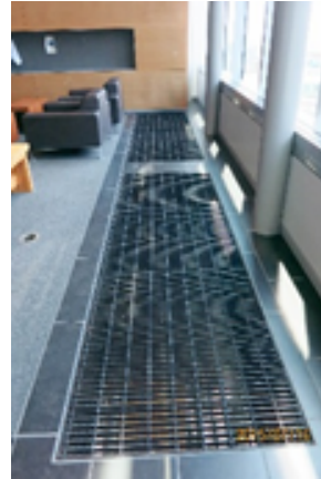
(b) Motorized floor grilles interconnect the atria
