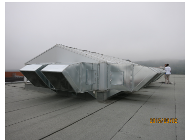
(d) Fans on the roof of the building assist ventilation
