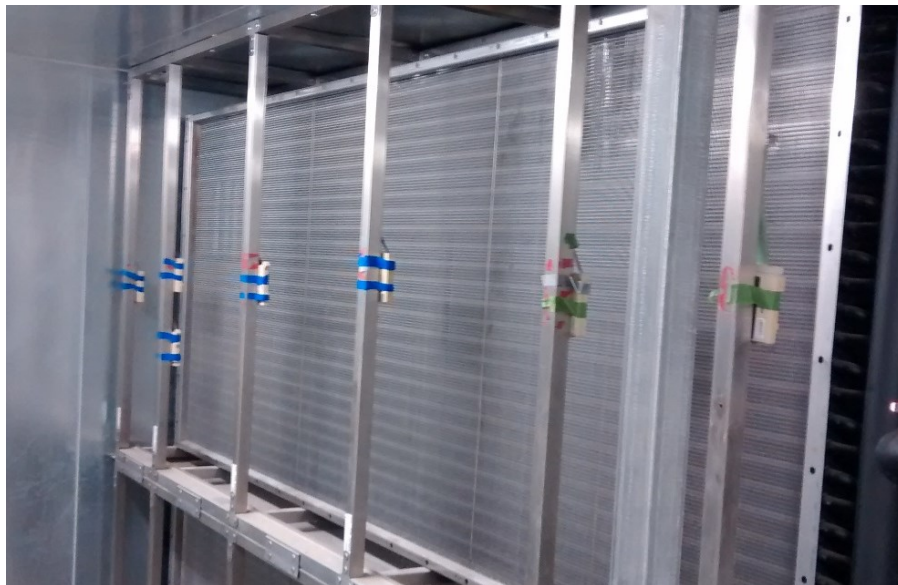
Figure 6.5 – Picture: air temperature portable sensors placed just after the heat recovery coil.
