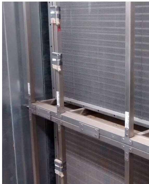
Figure 6.7 - Picture: air temperature portable sensors at different heights after the heat recovery coil while the heat recovery loop is not working.
