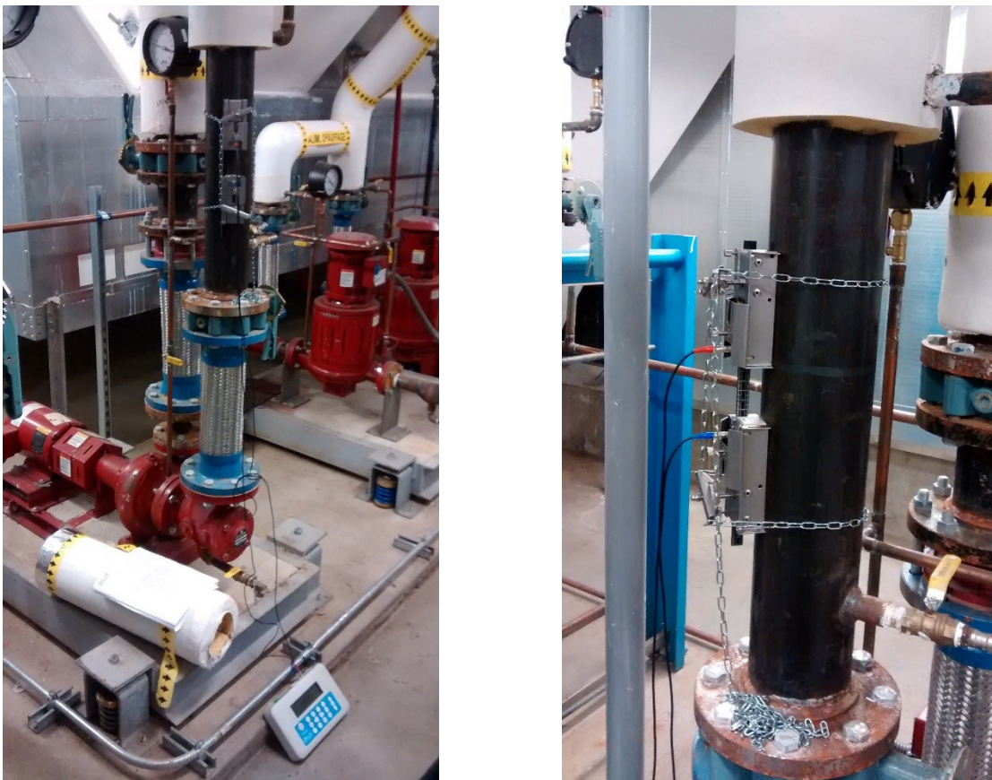
Figure 6.11 – Pictures of the portable flow meter installed just before pump P03-GLC.
