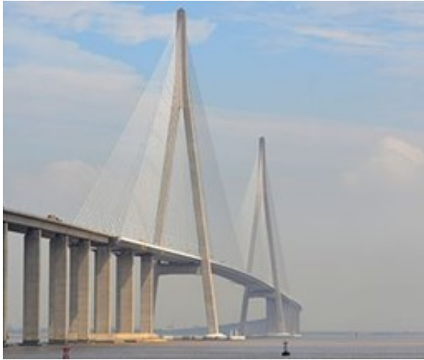
Figure 2-10 - Sutong Bridge ( Wikipedia )
