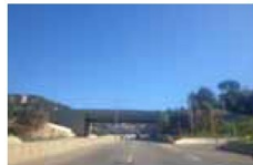
48- Jouret ElBallout Bridge 5
