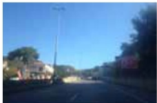
48- Jouret ElBallout Bridge 3
