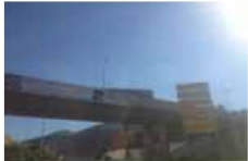
6- Nahrmot Baabdat Bridge 12
