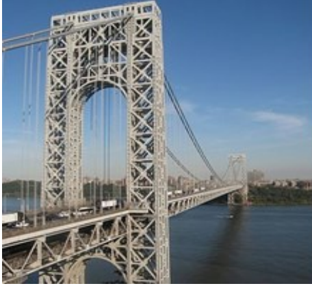
Figure 2-6 - George Washington Bridge ( Wikipedia )
