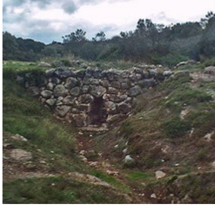
Figure 2-1 - Culvert of Arkadiko Bridge ( Wikipedia )
