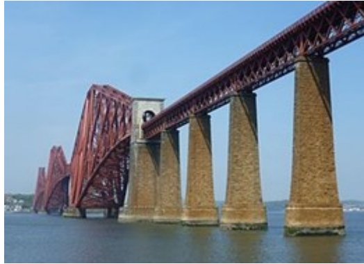
Figure 2-5 - Forth Rail Bridge ( Wikipedia )
