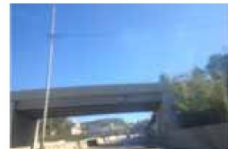
48- Jouret ElBallout Bridge 6
