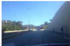
48- Jouret ElBallout Bridge 4
