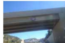
48- Jouret ElBallout Bridge 7
