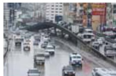
50- Jal-el-Dib Old Steel Bridge
