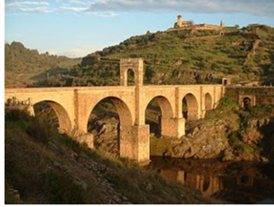
Figure 2-2 - Alcantara Bridge ( Wikipedia )
