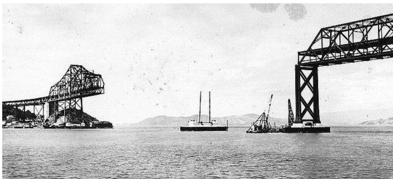
Figure 14 Frame grab from Lost Landscapes of San Francisco, 9 , San Francisco Bay Bridge during construction 1935 or 1936.
