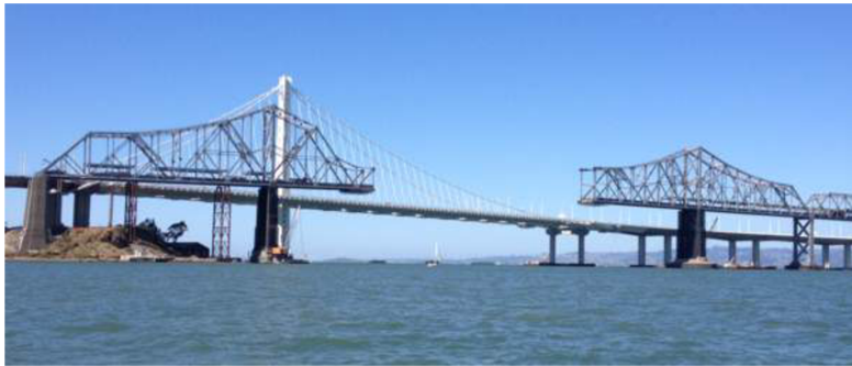
Figure 13 San Francisco Bay Bridge during demolition in 2014. Note the newly constructed bridge behind it.
