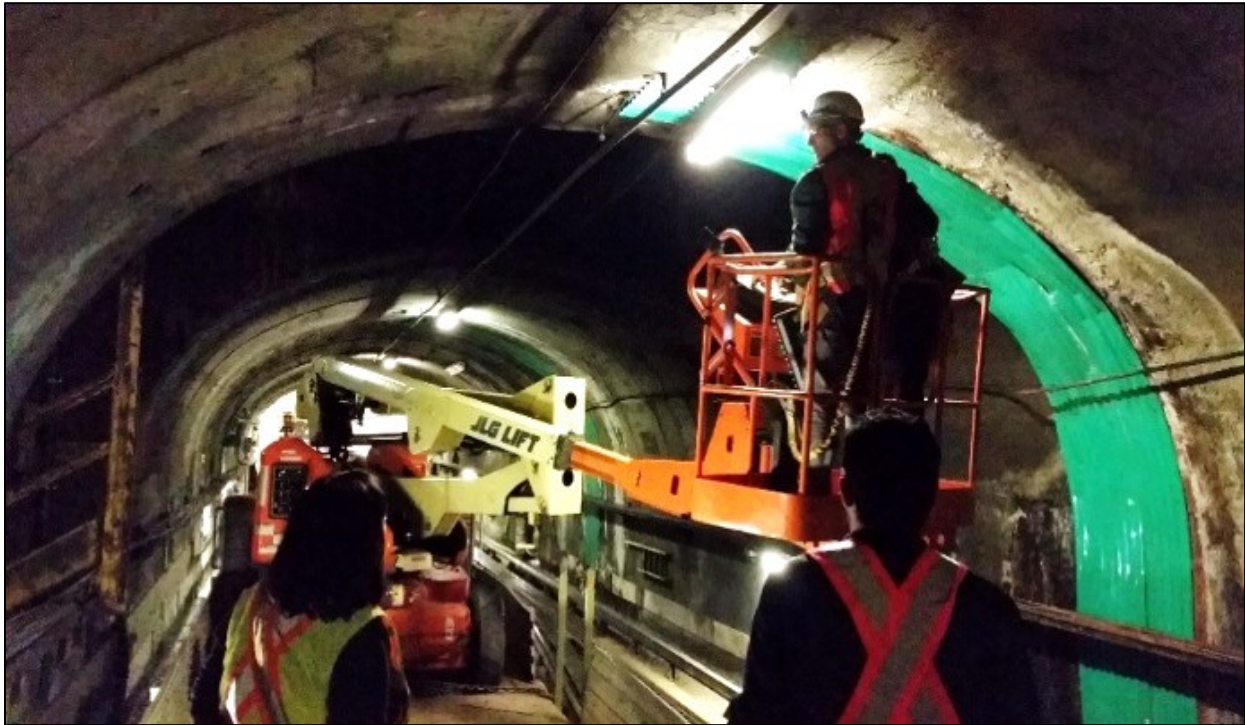
Figure 4.4 Image Acquisition Process in a Montréal Subway Tunnel (Dawood et al. 2017 a )
