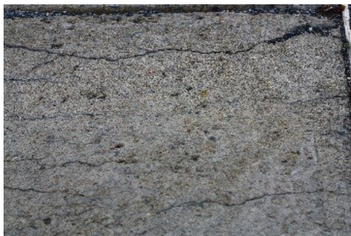
(a) Cracks on Lower Slab
