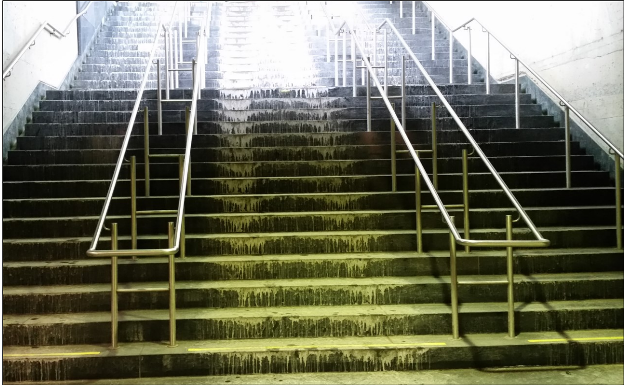
Figure 5.44 Salt on Stairs in a Montréal Subway Station
