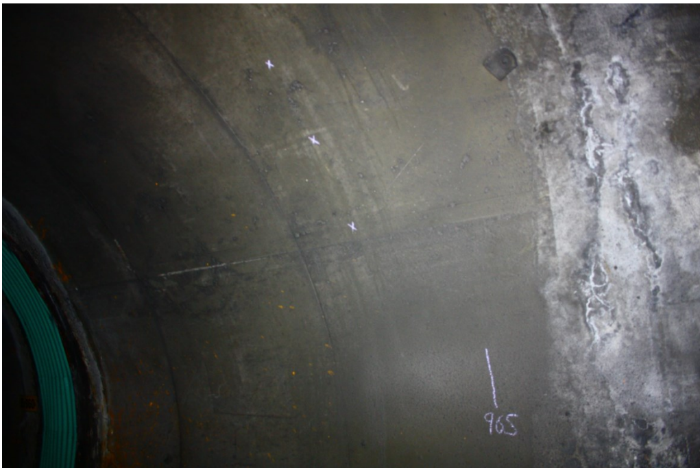
Figure A2 Marking Scanning Paths in the Tunnel Inter Frontenac and Papineau
