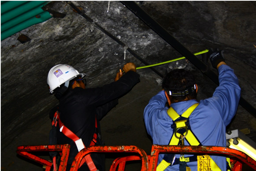
Figure A1 Measurements in the Tunnel Inter Frontenac and Papineau
