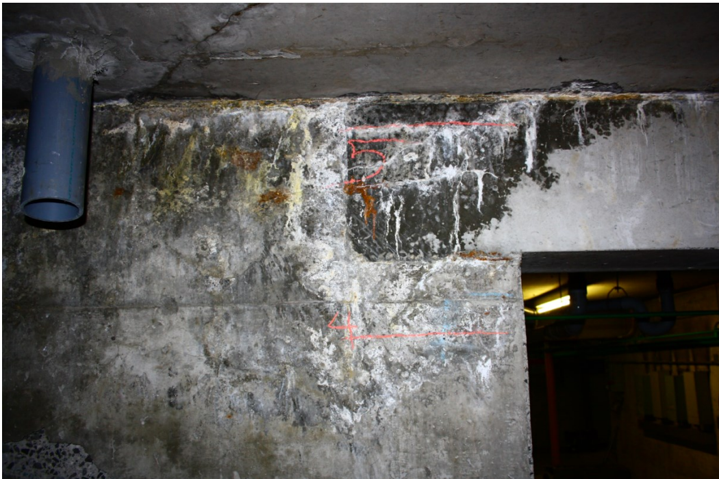
Figure A6 Marking Scanning Paths on a Wall in Outremont Station
