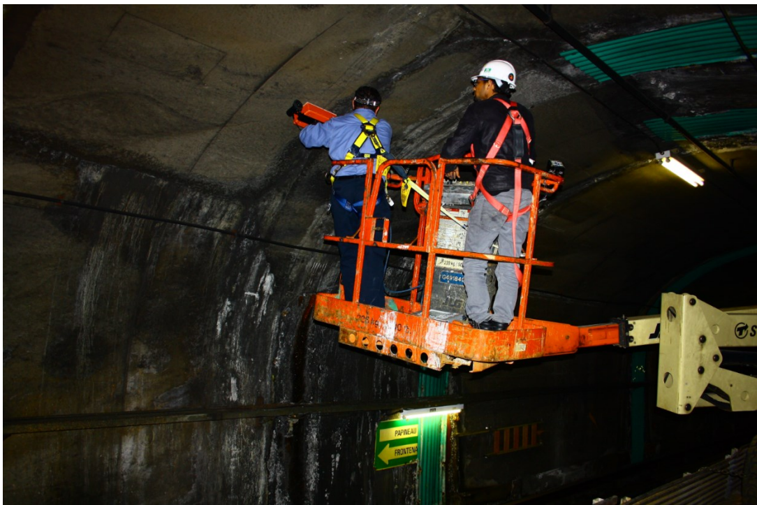
Figure A4 Scanning the Vault by GPR in the Tunnel Inter Frontenac and Papineau
