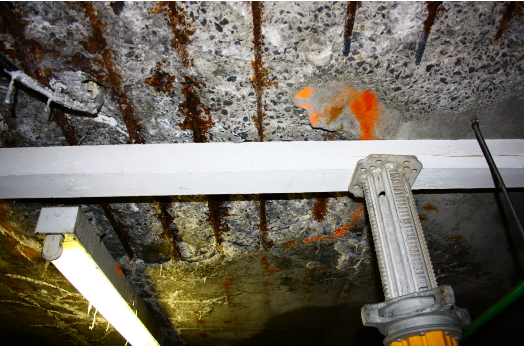
Figure A8 Corrosion, Delamination, and Efflorescence in Outremont Station
