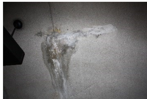
(b) Moisture Marks on Upper Slab
