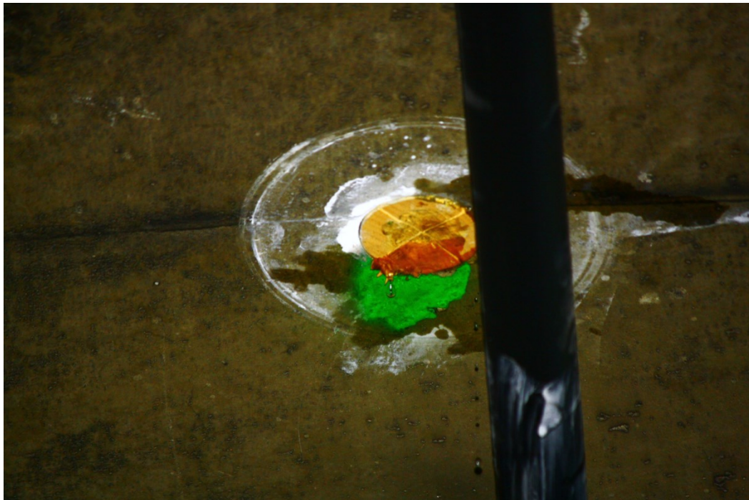
Figure A12 Dripping Water after Coring the Vault
