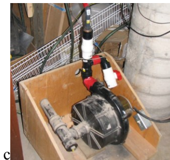
a) central air pump used for air injection
