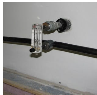
b) air injection port
