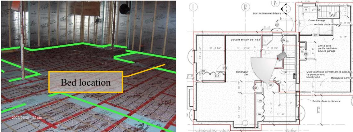
**Figure 45 : Heating Cables for SS-SDB, SS-SF and SS-CH1**
