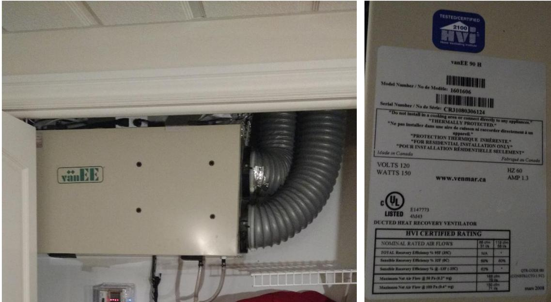
Figure 53 : Heat Exchanger Installation (Left) and Label (Right)
