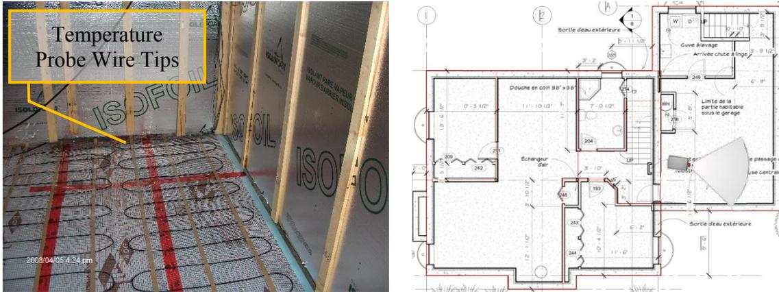
Figure 51 : Temperature Probes for SS-GAR-01 and SS-GAR-02
