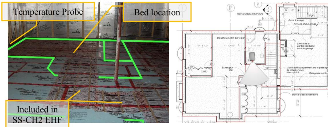
Figure 44 : Heating Cables for SS-CH2, SS-SF-STAIRS and SS-SF
