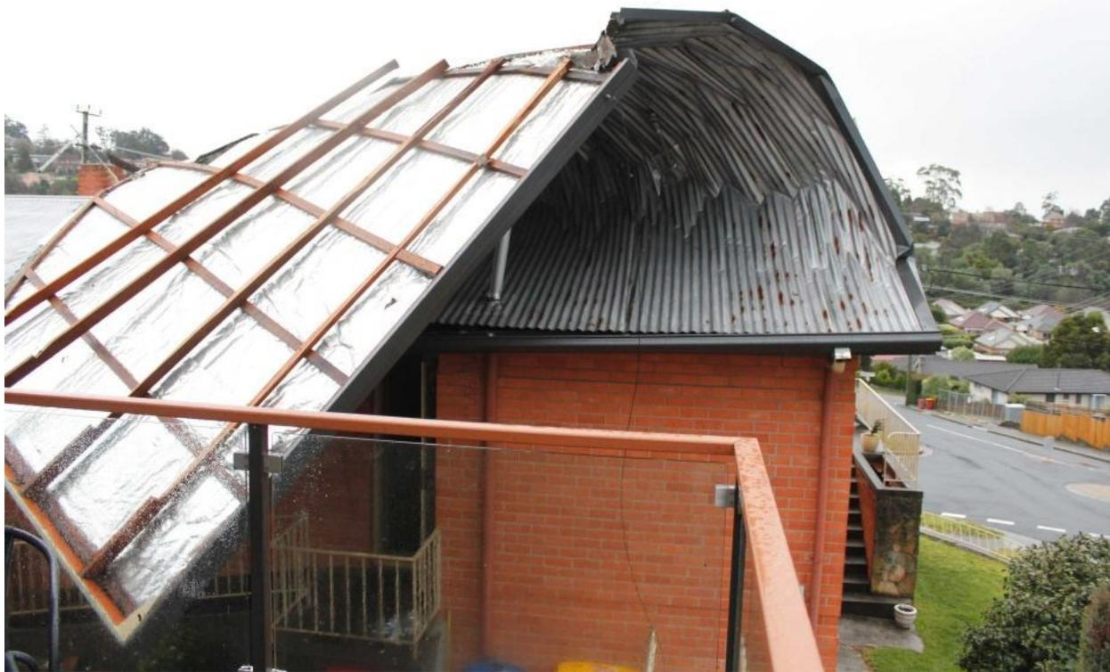
Figure 1-1: Roof damage of a new building due to a wind storm in Tasmania, April 2017 (<http://www.abc.net.au/news/2017-04-27/the-roof-peeled-back-from-a-house-in-kings-meadows/8475332>).
