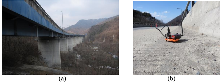
Figure 4.5 a) STB bridge details b) Data logger
