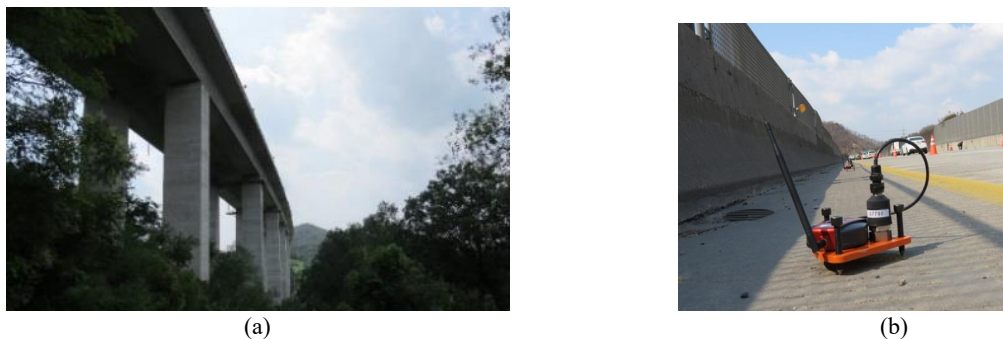
Figure 4.1 a) PSCB bridge details b) Data logger
