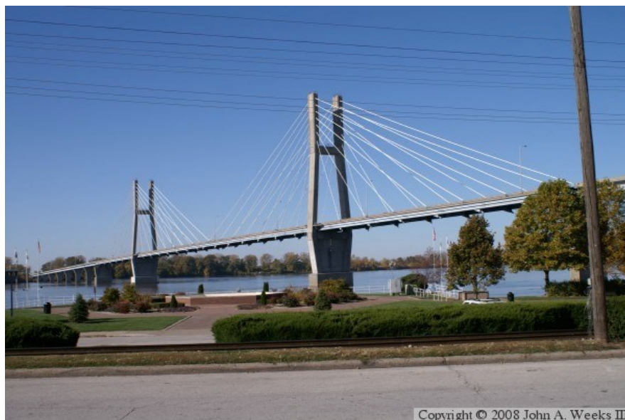
Figure 3.1 Quincy Bayview Bridge (Photo courtesy: John A.).
