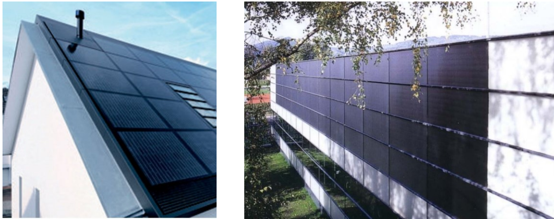
Figure 1.1: BIPV roof application (left) and solar collectors on the Meusburger Production Hall in Austria (right) (Weller et al., 2010; Zhang et al., 2015)
