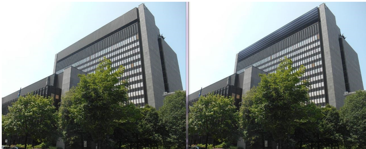
Figure 3.11: Actual south facade (left) and visualization of BIPV/T cladding at penthouse level of the facade (right)
