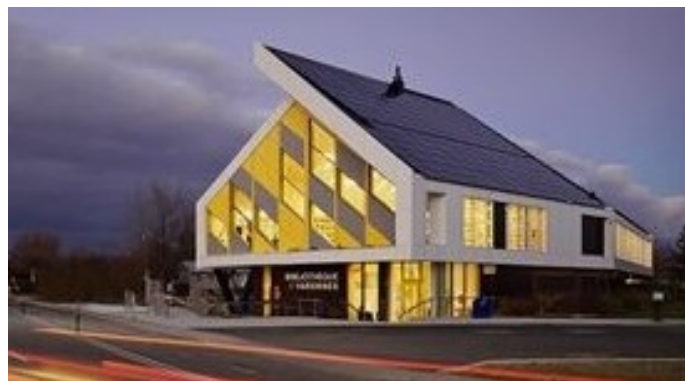
Figure 2.8: The BIPV/T roof of the Varennes library in Varennes, Quebec
