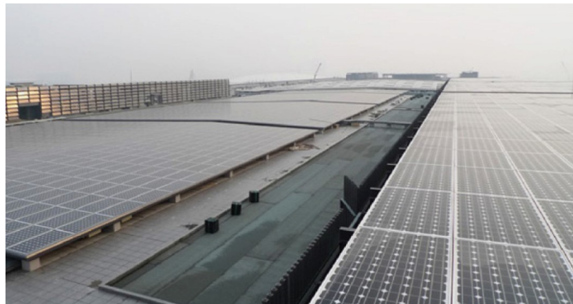
Figure 2.2: Installed BAPV system (Peng et al., 2011)
