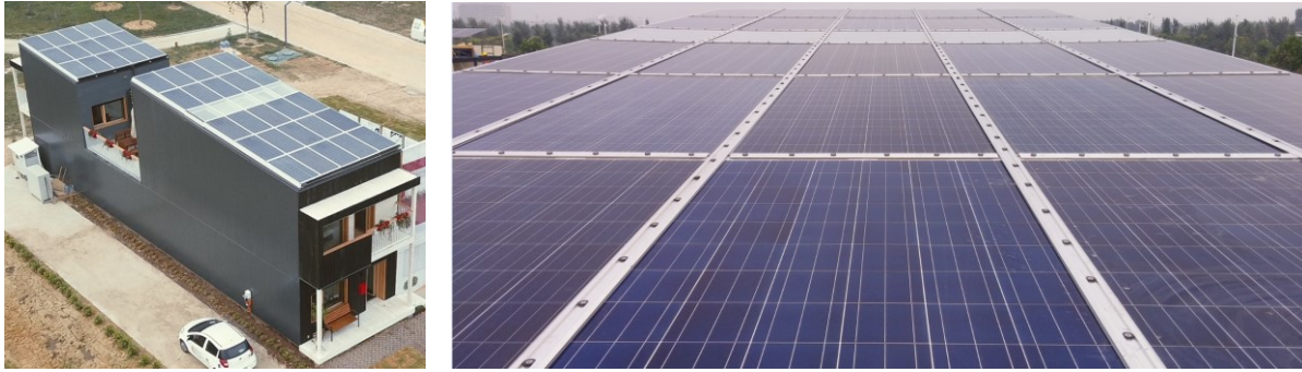
Figure 3.16: Deep Performance Dwelling aerial view (left) and BIPV/T roof after completion (right) (Rounis et al., 2017)
