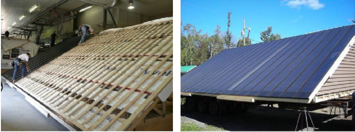
Figure 2.7: Wood sub-framing for roof at factory (left) and BIPV/T finished module on-site (right) (Chen et al., 2010)
