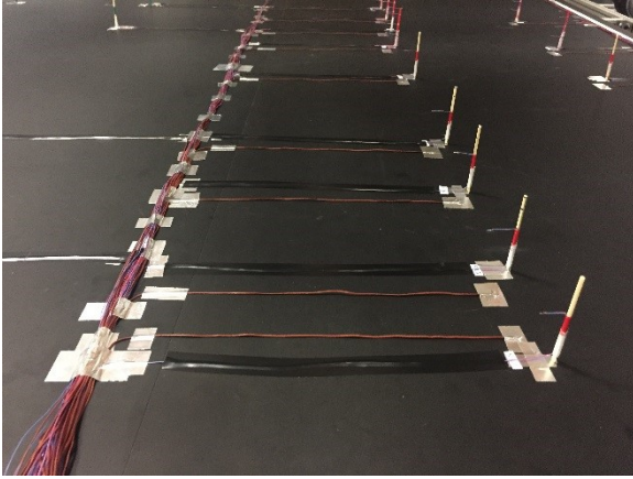
Thermocouples installed over insulation and absorber in channel
