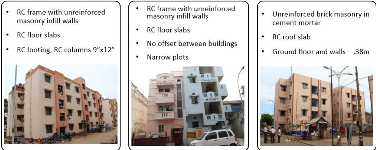
Figure 3.21: Building typologies in the state of Tamil Nadu (National Disaster Management Authority, 2013)
