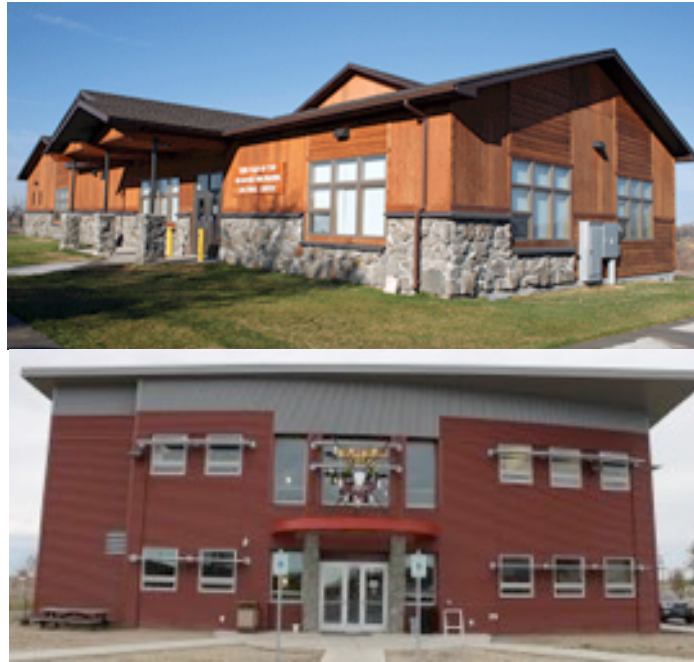
Figure 5: Buildings from the Aaniiih Nakoda College (Fort Belknap, from their Website)
