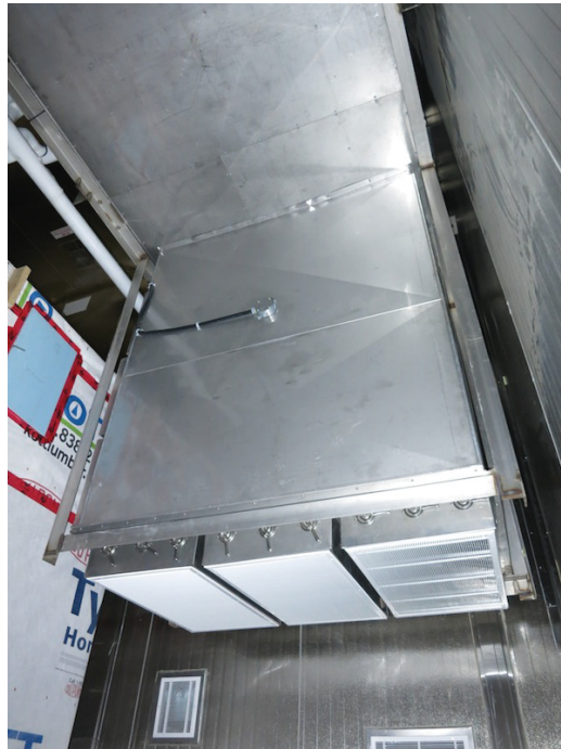
Figure 3.8 HVAC system air supply in the environmental chamber
