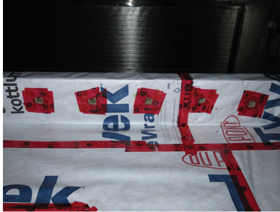
Figure 3.7 vents in soffit of ventilated attic
