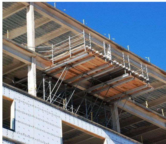
Figure 6 Example of Cantilever Scaffolding [16]
