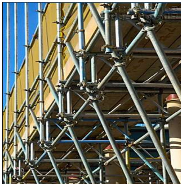
Figure 2 Example of tube and clamp Scaffolding [12]
