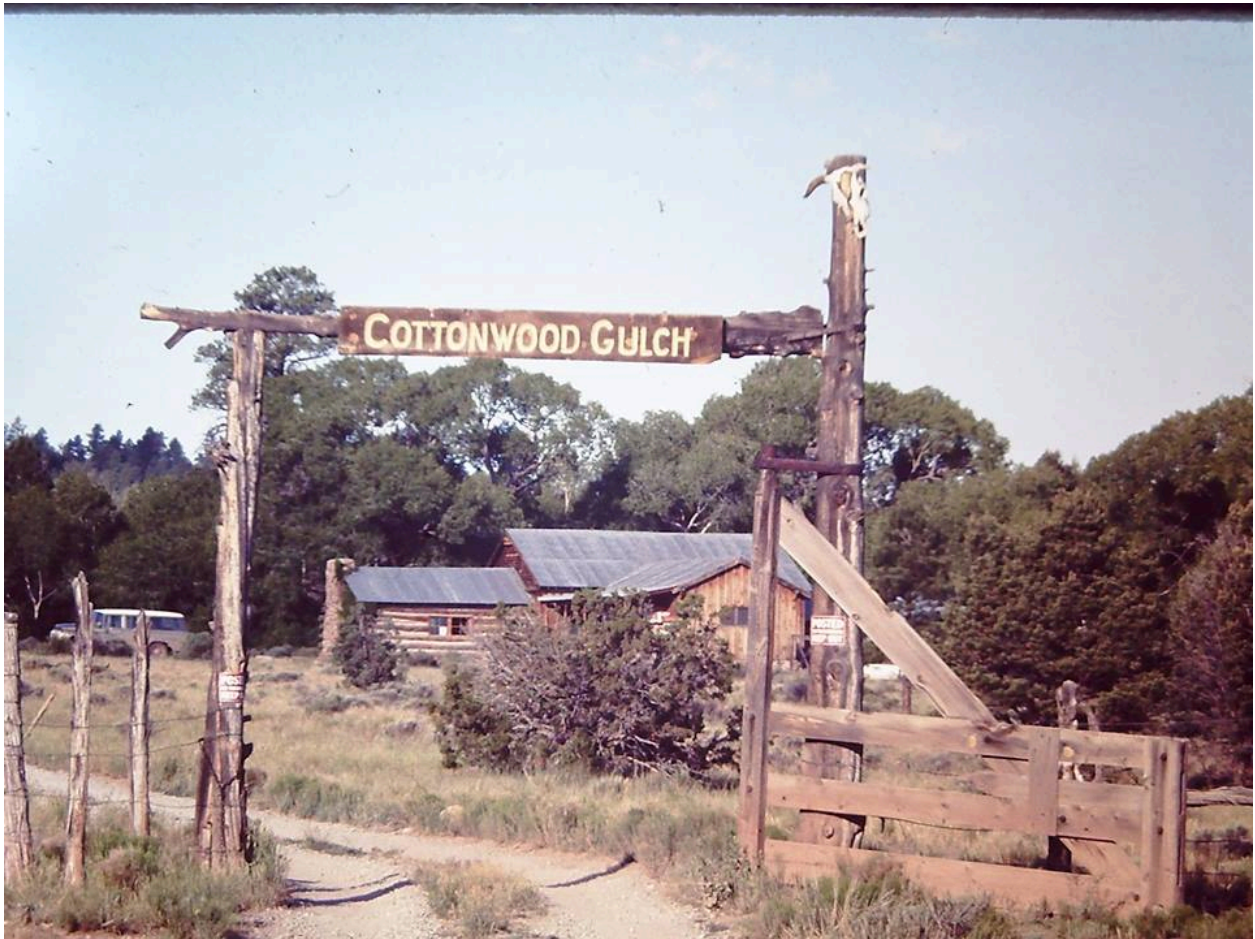
Figure 10: Entrance to Basecamp. Photo courtesy of Cottonwood Gulch.
