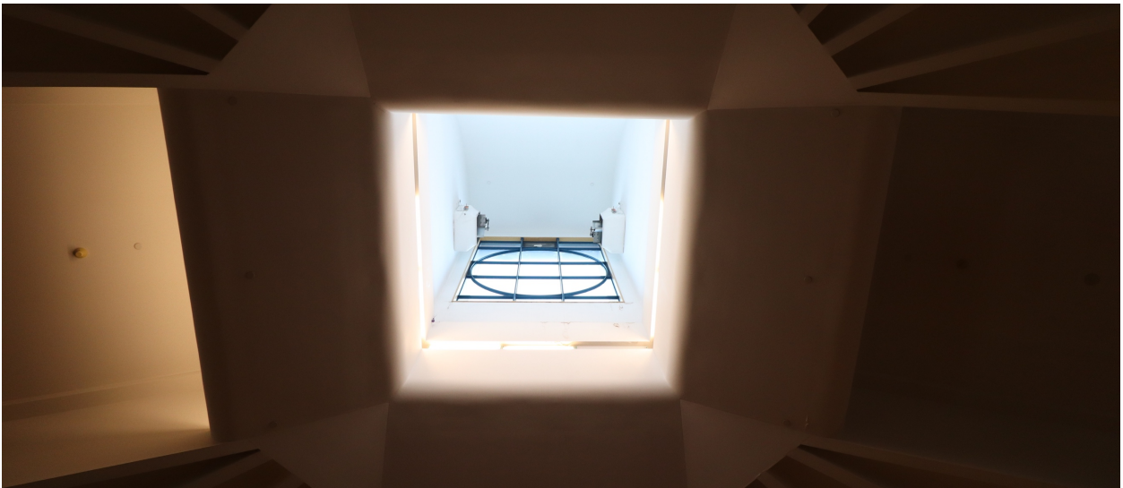
Figure 29 – Douglas Cardinal, Motorized window and ventilation system, interior view, Circle of Life Thunderbird House (2001), Winnipeg, Manitoba. Photo by Gabrielle Montpetit, taken October 9, 2018.
