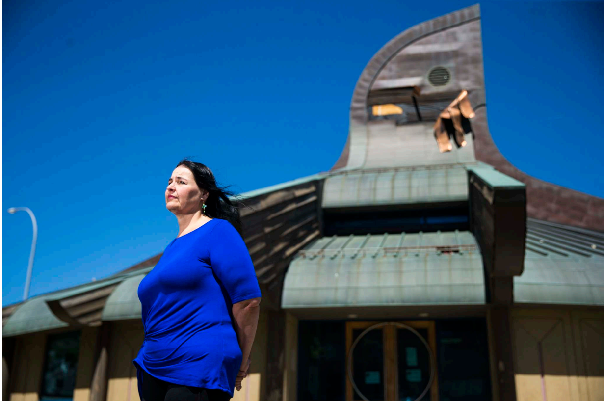
Figure 24 – Richelle Scott, former co-chair of Circle of Life Thunderbird House Board of Directors, standing in front of Circle of Life Thunderbird House and the copper plates falling off the roof. Photo by Mikaela Mackenzie. Image Source: Ryan Thorpe. “Thunderbird House Pleas for Help Ignored, Board Co-chair Says.” Winnipeg Free Press , July 11, 2018. https://www.winnipegfreepress.com/local/thunderbird-house-pleas-for-help-ignored-board-co-chair-says-487825571.html .
