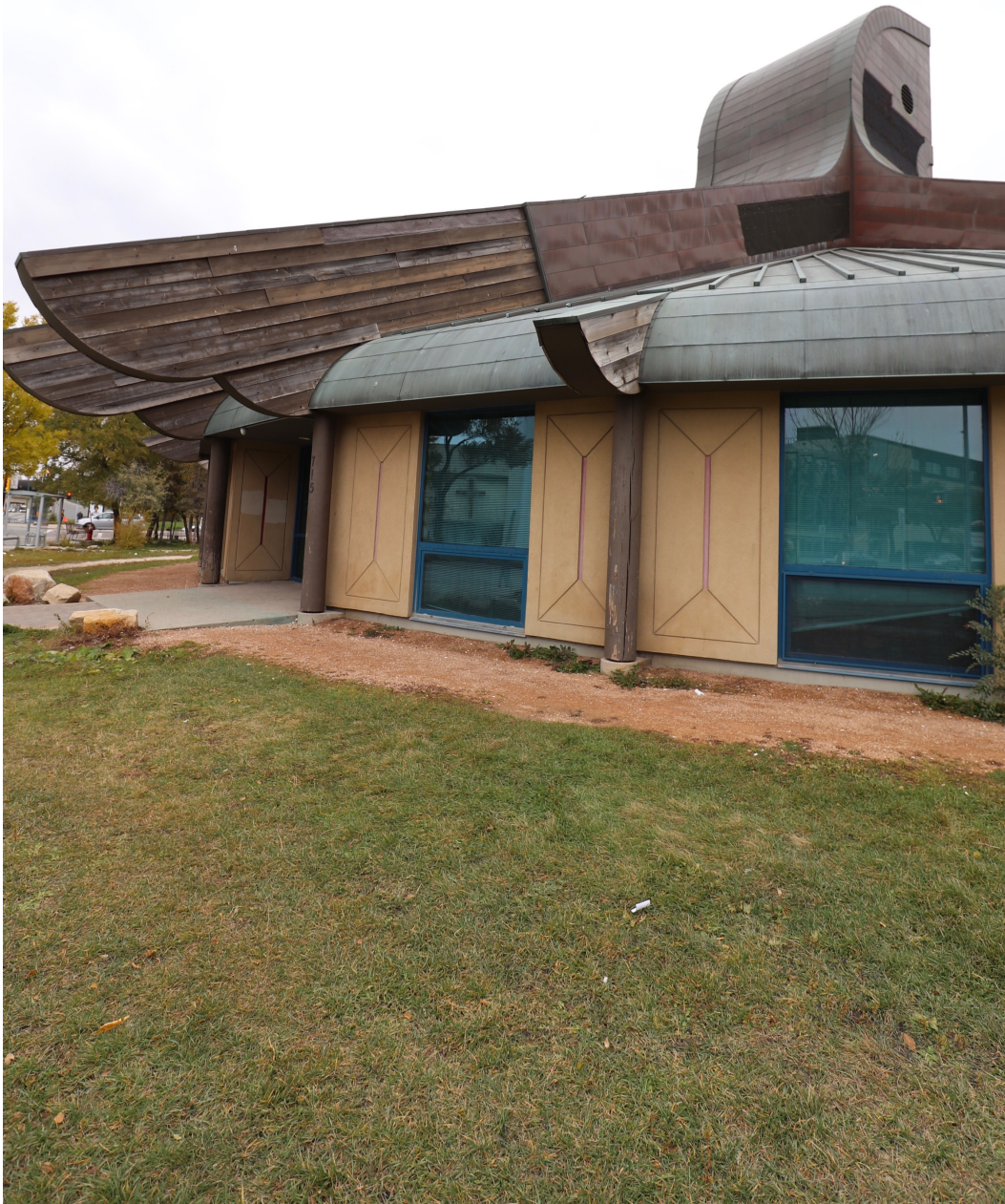
Figure 23 – Douglas Cardinal, Roof detail, Circle of Life Thunderbird House (2001), Winnipeg, Manitoba. Photo by Gabrielle Montpetit, taken October 9, 2018.
