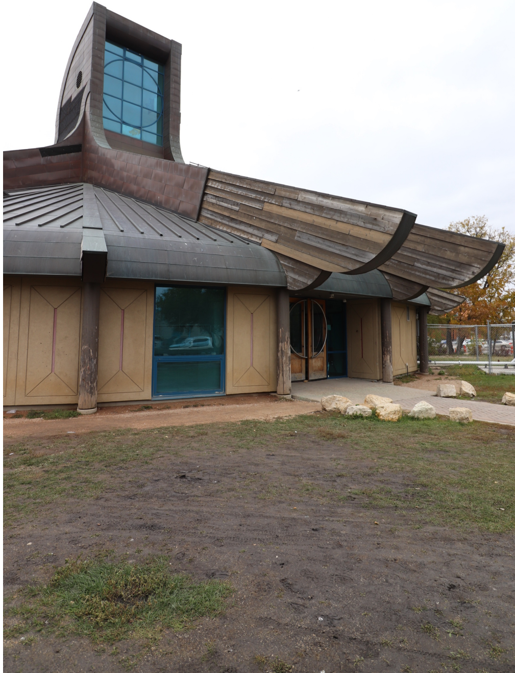
Figure 25 – Douglas Cardinal, Roof detail, showing skylight, Circle of Life Thunderbird House (2001), Winnipeg, Manitoba. Photo by Gabrielle Montpetit, taken October 9, 2018.
