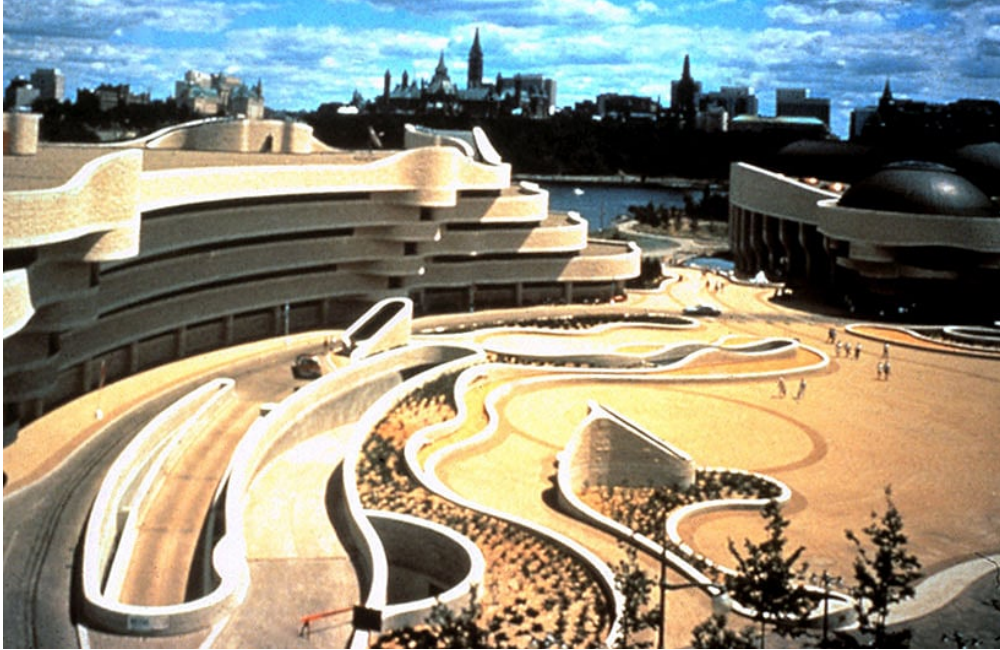
Figure 4 – Douglas Cardinal, Museums of Civilization (now the Canadian Museum of History) (1989), Hull, Québec. Image Source: Douglas Cardinal Architect, Museum of History, accessed June 27, 2019, http://www.djcarchitect.com/work#/museum-of-history/ .
