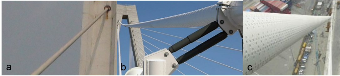
FIGURE 1-1 THREE TYPES OF CABLES: A) REGULAR CABLE 1 , B) CABLE WOUND WITH A SPIRAL WIRE 2 , AND C) DIMPLED CABLE 3
