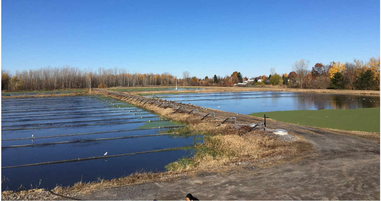
Figure 4: Four lagoons in the City of L'Assomption WWTP
