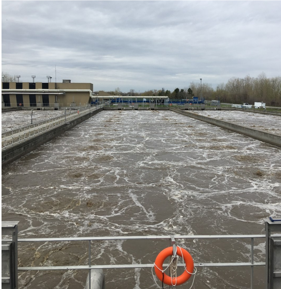
Figure 6: Activated sludge reactor in the City of Saint-Catherine WWTTP, where the sludge was brought from
