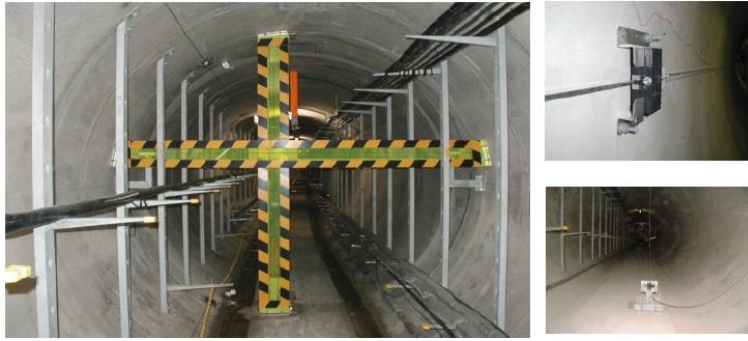
Figure 2-11: Optical fiber sensor in a MUT (Nakano et al., 2011)
