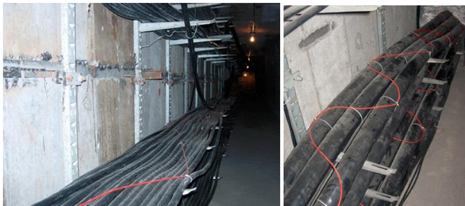
Figure 2-16: Temperature sensors for cables (Senkox, n.d.)
