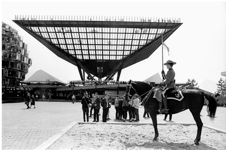
Exterior view of the Canada Pavilion with RCMP officer on guard, Expo 67, Montreal
