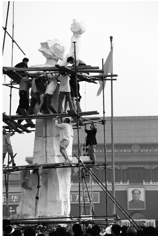
Construction of the Goddess of Democracy in Tiananmen Square, 1989
