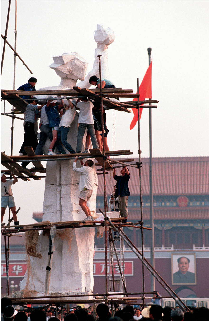
Construction of the Goddess of Democracy in Tiananmen Square, 1989
