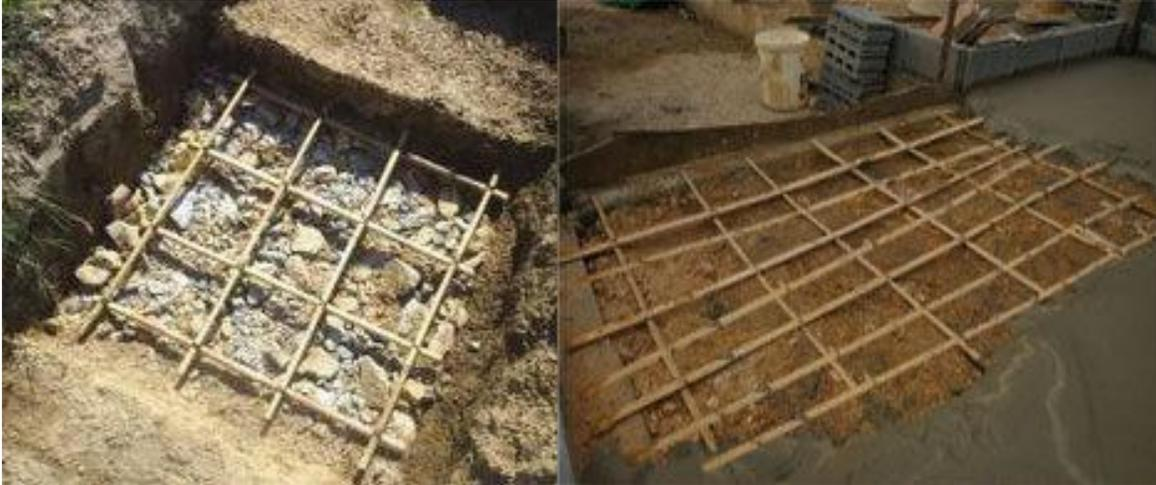
Figure 2.4 Bamboo as Reinforcement [85]
