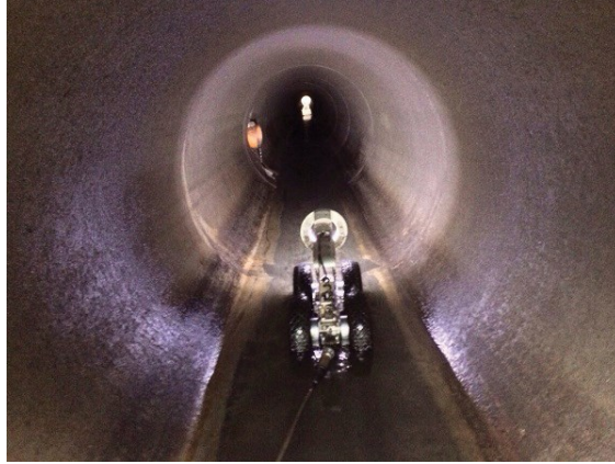
Figure 2-12. CCTV inspection for sewer pipeline.
