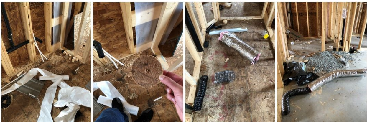
Fig. 2: Construction waste produced during MEP system installation
