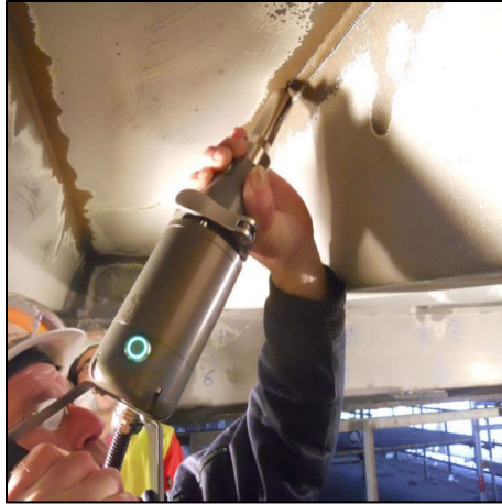
Figure 24: Detecting of a fatigue crack initiation followed by preventive treatment
