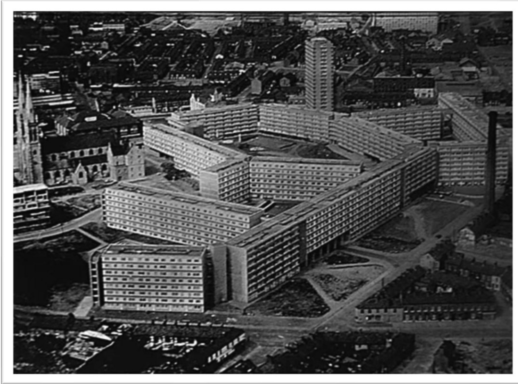
Figure 13. Aerial view of the Divis Flats. Architect Frank Patterson. Photographer unknown. sourced from ArchiSeek: https://archiseek.com/2014/1969-divis-flats-belfast-co-antrim/ Accessed May, 16, 2020.
