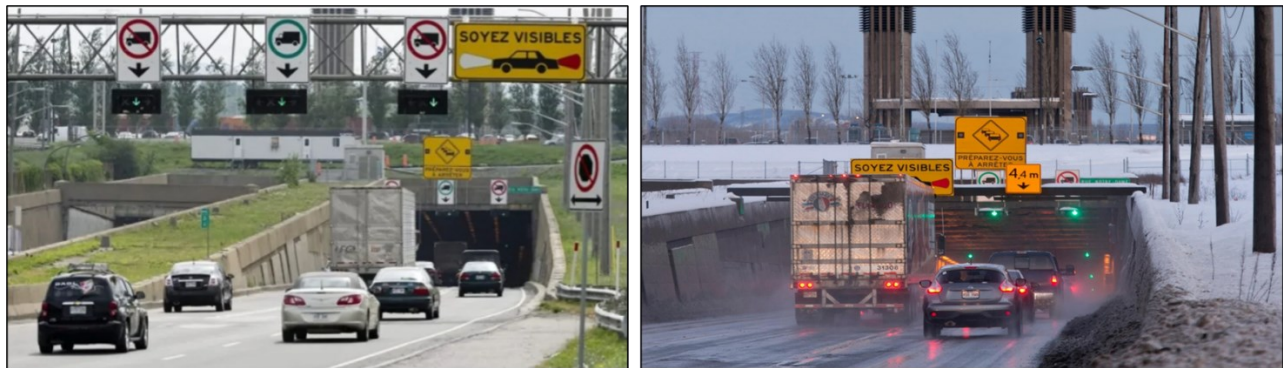
Figure 0-1. LHL tunnel in different seasons 10
