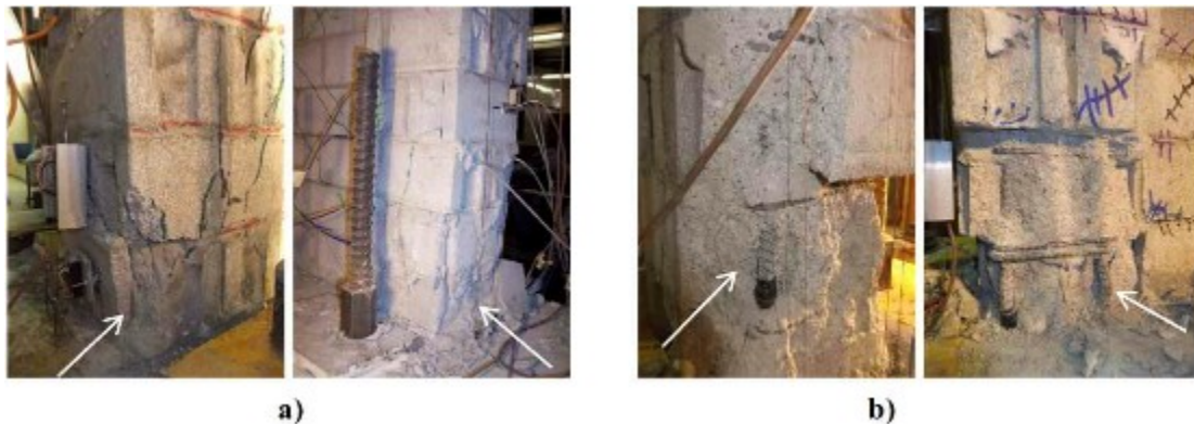
Figure 2.4 Visually observed damage states: (a) Spalling of the face shell and vertical cracking; (b) crushing of the masonry (Banting 2013)
