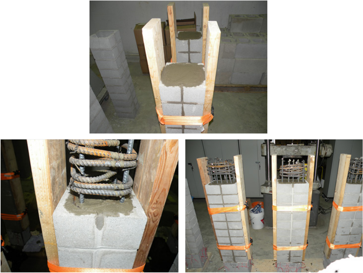
Figure A.14 Grouting of unreinforced MBE prisms and RMBEs
