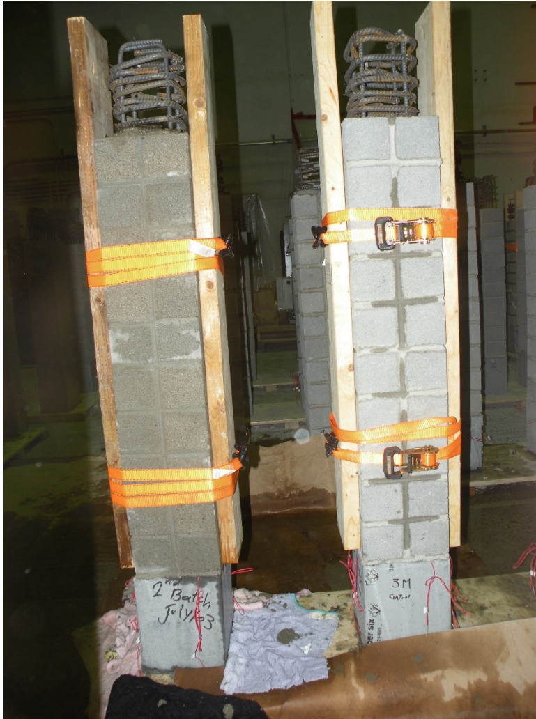
Figure A.13 Dry and wet RMBEs before grouting
