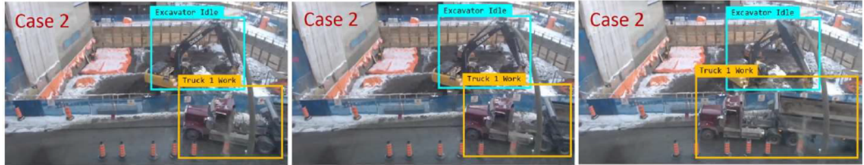
(b) Case 2: Excavator is waiting for truck maneuvering
