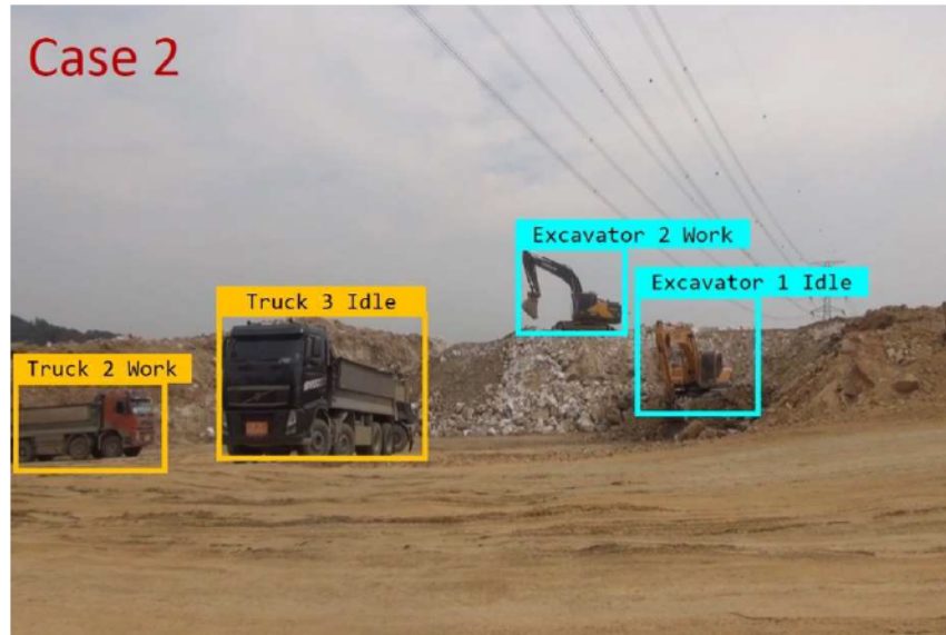
Figure 5-13 Example of trucks' occlusion (Case Study 2)
