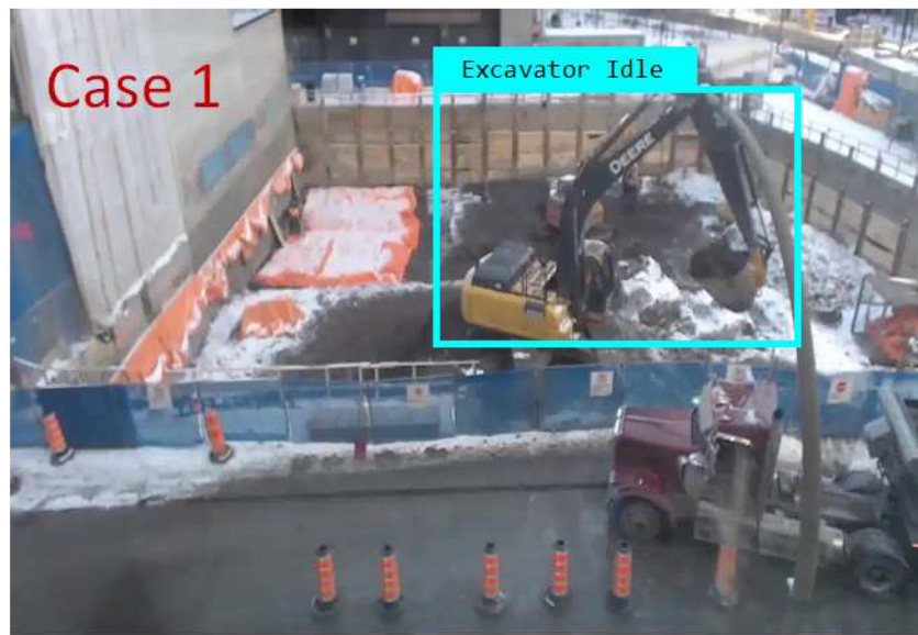
Figure 5-6 Example of lost detection for the partial truck (Case Study 1)
