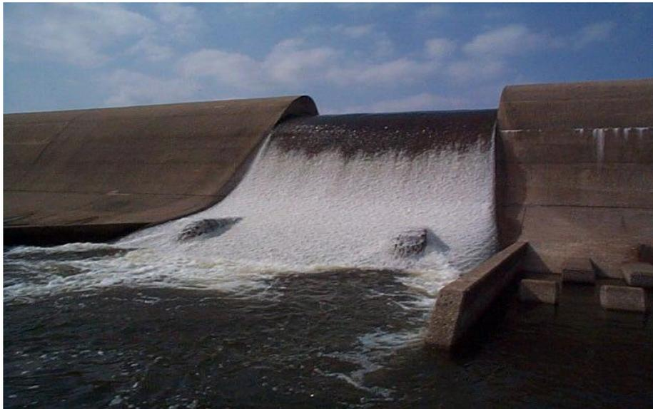
Figure 1-4. Longitudinal profile of ogee spillway (from Nalluri and Featherstone, 2009), and photo of Rend Lake Spillway, Illinois, U.S. (<https://www.pinterest.ca/pin/68609594297759152/>)
