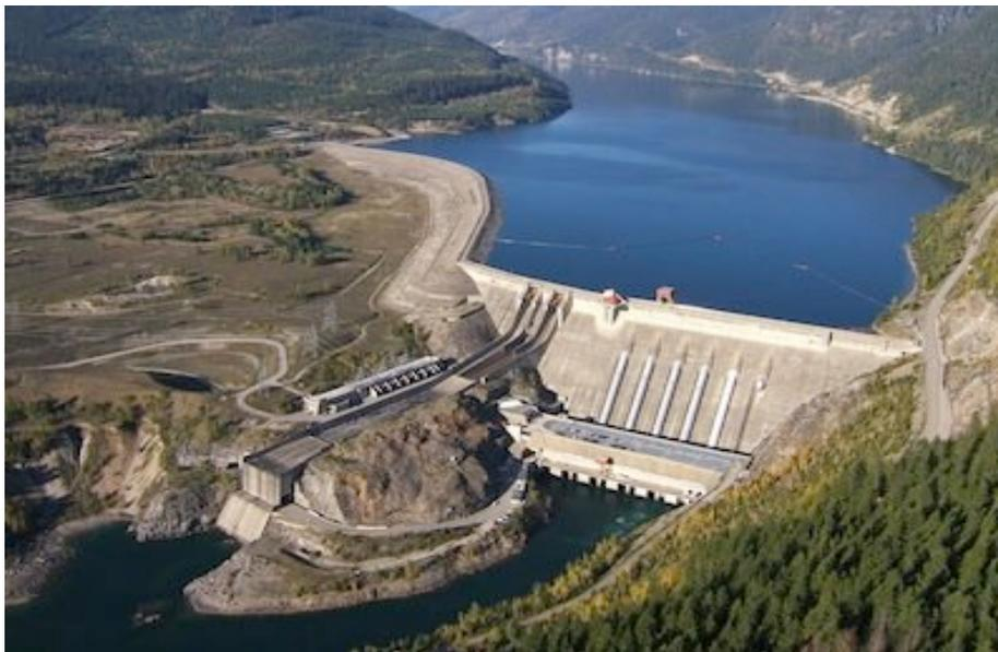
Figure 1-5. Side channel spillway (Houghtalen et al., 2017) and photo of Revelstoke side channel spillway, Revelstoke, B.C., Canada (<https://www.pinterest.ca/pin/54817320442348907>)
