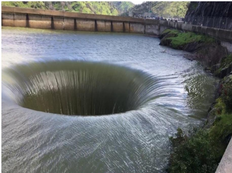
Figure 1-2. Trough spillway (<http://hydropedia.blogspot.ca/2014/03/spillway.html>, accessed on June 1, 2017) and photo of Glory Hole Spillway at Lake Berryessa, California, U.S. (<https://www.usbr.gov/newsroom/stories/detail.cfm?RecordID=58763>)
