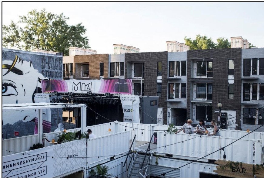
Figure 3.17: A new condominium complex under construction over an old parking lot next to Mural Festival VIP area. 2017. Photo by Kris Murray.
