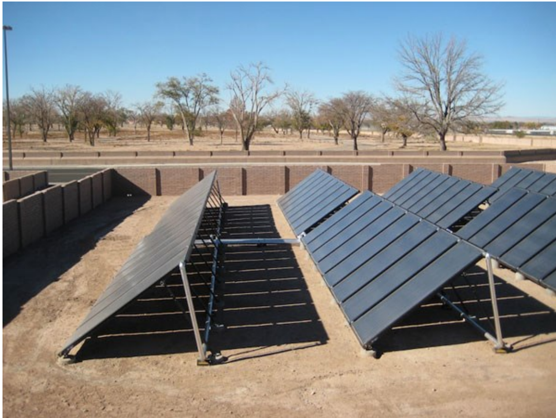
Figure 33 Solar collectors' installation (source from:
