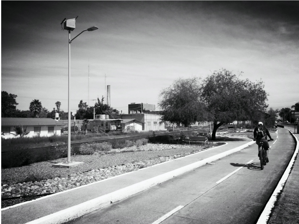
Figure 63. Missing solar charger for light, Ciclovía Gómez Morín. Photo by author
