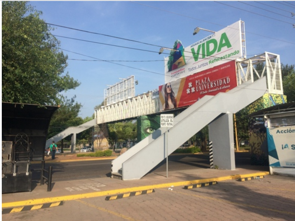
Figure 42. One of many so-called pedestrian bridges in Aguascalientes. With the exception of four new overpasses with elevators, the vast majority of these bridges in Aguascalientes are accessible only via concrete stairways, posing major accessibility challenges for cyclists and many pedestrians. In light of these issues, the term “anti-pedestrian bridge” was coined by Mexico’s Liga Peatonal (Pedestrian League) to refer to overpasses that privilege rapid motor-vehicle traffic while creating an uninviting and often unsafe space for active travelers 120 Photo by author
