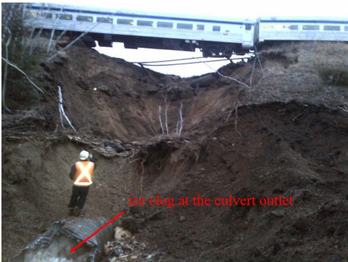
Figure 1.2 Ice blocking culvert outlet (TSB 2013)
